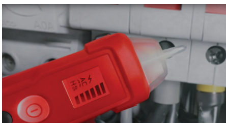
Verification of voltage presence on outlets, terminals, cables, and equipment
